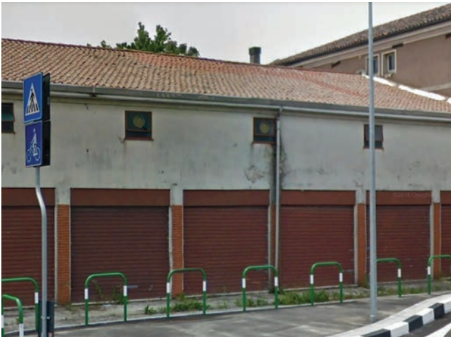
The building in Padova, Italy where Hanna Instruments was founded.
